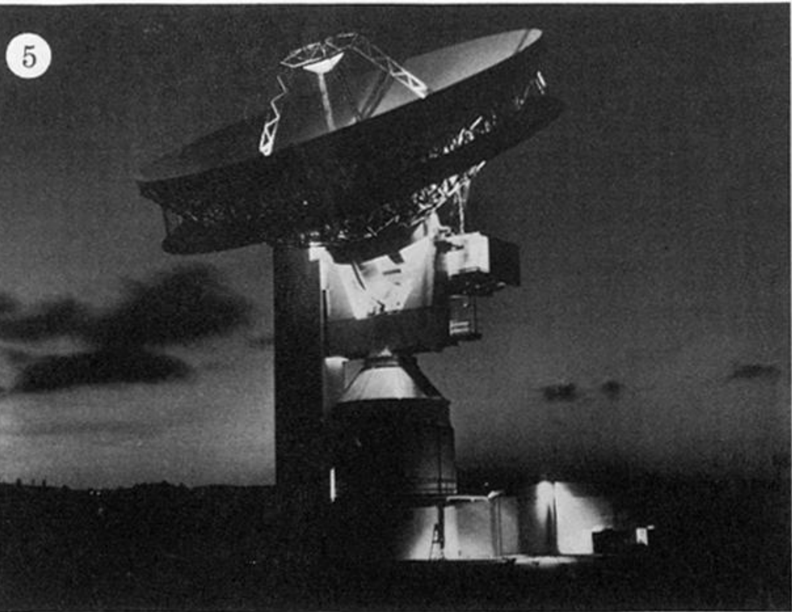
FIGURE 5. Antenna at Etam, West Virginia.
