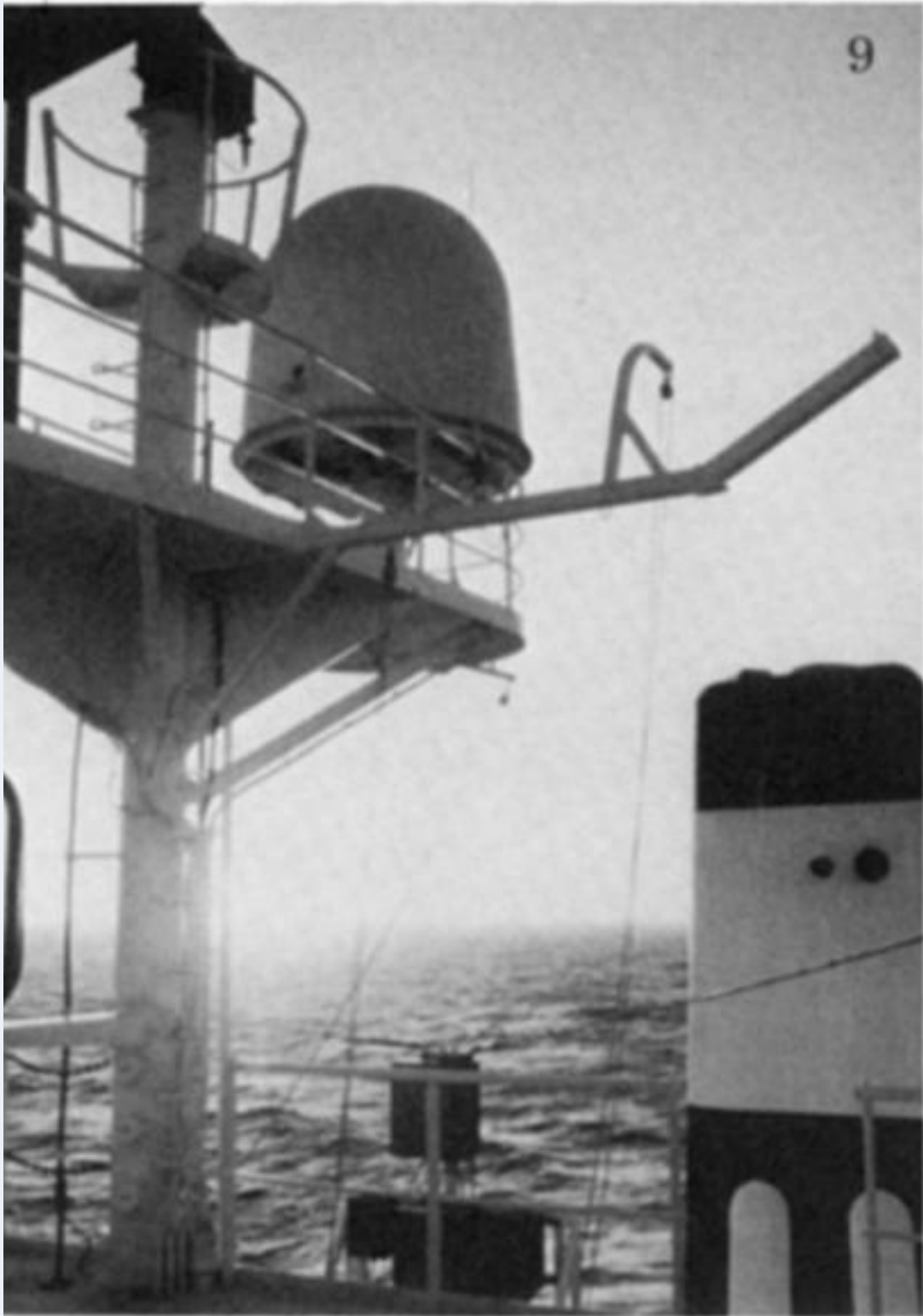
FIGURE 9. A maritime installation.
